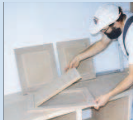
The author made the raised-panel doors from two pieces of MDF — one for the frame and one for the panel (above). The radiused corners left in the frame by the router were squared with a chisel (left). The panel profile was cut with a table-mounted router.
