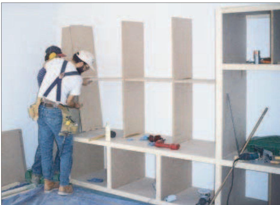
Figure 2. With the tall carcass in place, the rest of the panels were installed piece by piece. Unlike shop-built cabinets, which require a back panel for stability, a built-in can use the existing house wall for support.
