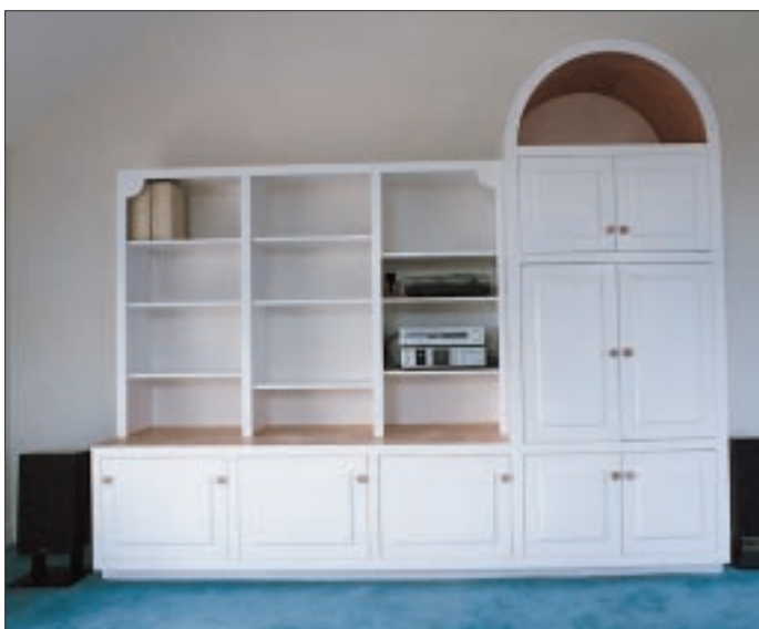
Figure 3. The author cut the curved frame and face trim for the vaulted top of the cabinet with a jig-piloted router (left), then skinned the assembled vault with bending plywood (above). The finished vault mounted easily into place with screws.
