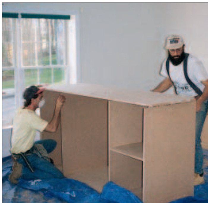
Figure 1. The author cut the cabinet panels to rough size in his shop, then scribed each piece of the carcass to the wall (far left). The two-man crew assembled the tall carcass on the floor before setting it into place (left).
