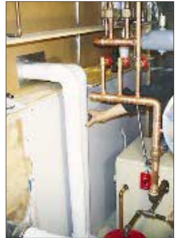
Plastic vent pipe joints should pass a 100-lb. pull test, but end-point connections must allow for expansion and contraction.
