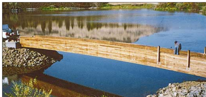
A new high-strength, lightweight glulam, used here to support a pedestrian bridge, incorporates a layer of fiber-reinforced plastic.
