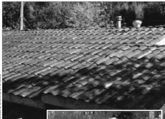
Durable tire roofs are a recycling solution that's guaranteed for 50 years or 100,000 miles.
