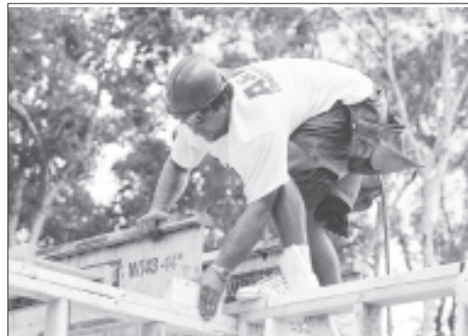
A uniform spec for I-joists would eliminate differences that make it hard to order and use engineered lumber.
