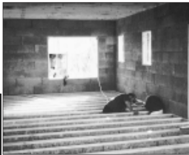
Wood I-joists, fly-ash concrete blocks, and a heat-reflecting radiant barrier helped earn green points for this low-budget home in Austin, Texas.
