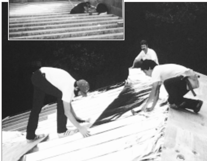
Wood I-joists, fly-ash concrete blocks, and a heat-reflecting radiant barrier helped earn green points for this low-budget home in Austin, Texas.
