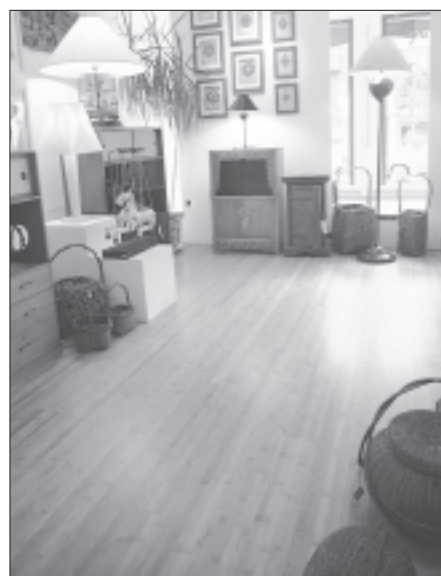
"Plyboo" bamboo flooring, which is nearly as hard as oak and can be sanded and finished like any wood flooring, has a tawny blonde color and a unique grain.
