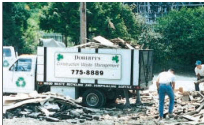
Construction Waste Management employees sort and haul away recyclable debris on a Seattle-area job site.
