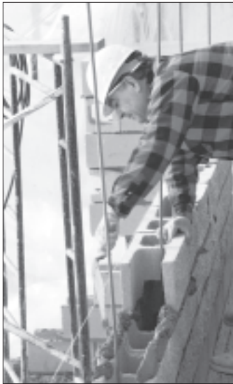
Skilled masons have no trouble with Integra's unusual block shape (left), but foaming the completed walls (above) requires a specially trained crew.
