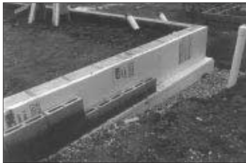
Rigid foam insulation board can protect shallow footings from frost action in northern climates.
