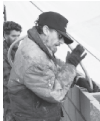
Skilled masons have no trouble with Integra's unusual block shape (left), but foaming the completed walls (above) requires a specially trained crew.
