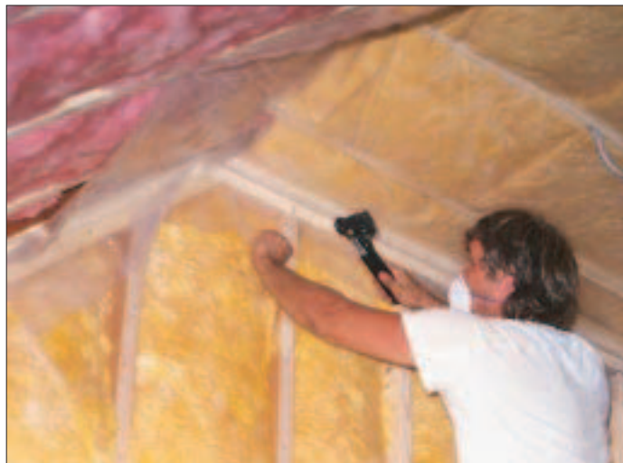
Figure 2. Loose-fitting fiberglass batts (left) will reduce the overall performance of a wall or ceiling system; a snug fit and a carefully installed air/vapor barrier ensure that the batts will yield close to advertised R-value (right).
