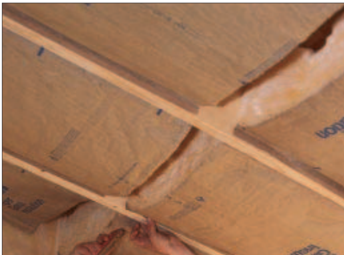
Figure 2. Loose-fitting fiberglass batts (left) will reduce the overall performance of a wall or ceiling system; a snug fit and a carefully installed air/vapor barrier ensure that the batts will yield close to advertised R-value (right).
