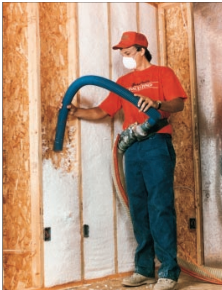
Figure 3. The fiberglass-based Blown-In-Blanket system provides an effective air barrier and an insulating value of R-4 per inch. The installer blows loose fiberglass mixed with a latex binder behind a nylon netting stapled to the face of the framing.
