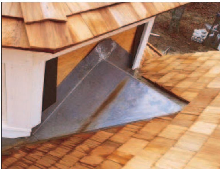
Figure 7. A cricket should be a single piece of metal, whether shop-fabricated or soldered together on site. To permit expansion and contraction, attach a cricket with cleats.
