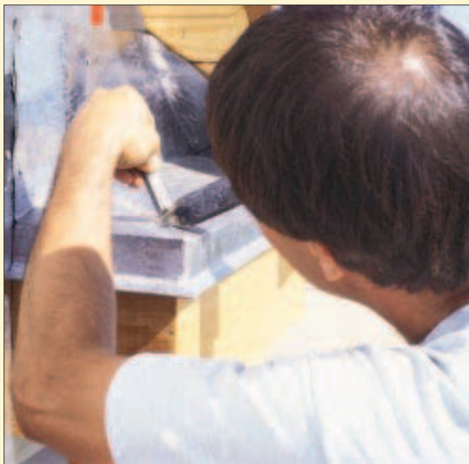
For extra strength, the author first joins large pieces of metal with a flat lock seam, then solders the joint (left). When soldering, heat the joint with the iron, then touch the solder to the heated metal (right).
