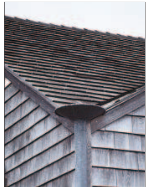
Figure 6. The author catches water at the junction of two cross gables with a soldered, cone-shaped scupper. Besides being attractive, the cone lets excess water spill over rather than backing up beneath the roof.
