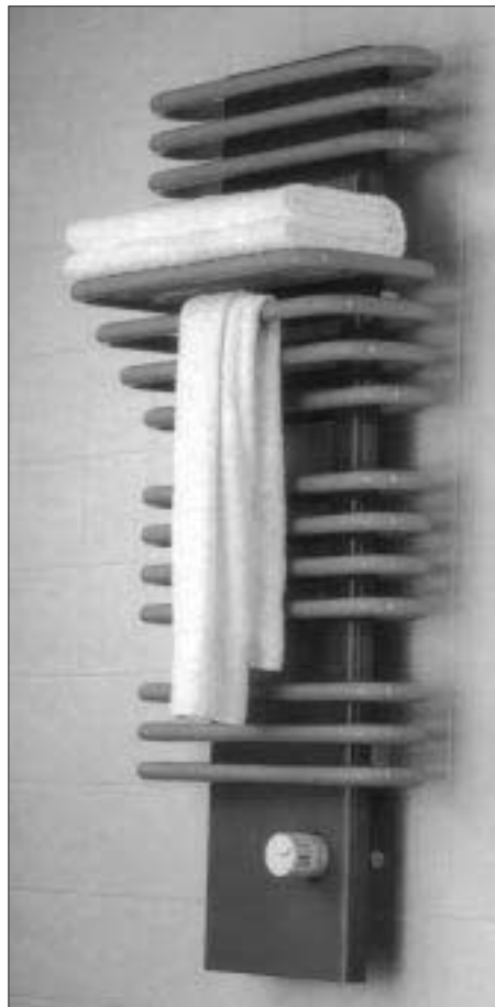
Figure 3. High-tech panel radiators are everywhere, while fin-tube baseboard is nonexistent. This radiator and towel warmer has a built-in thermostatic valve — a common zone control for European hydronic systems.
