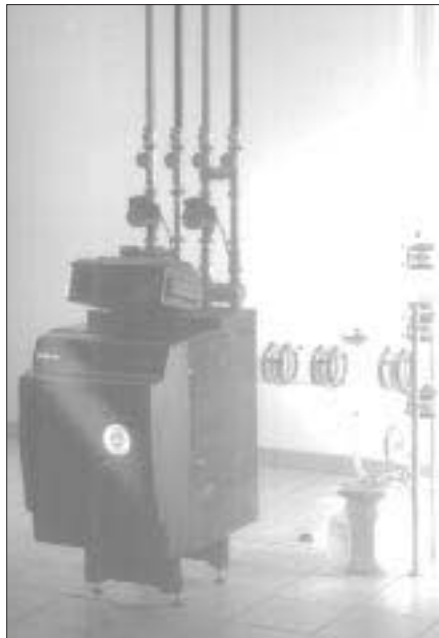
Figure 1. Condensing boilers that run at 95% efficiency are not uncommon in Europe, but the acidic condensate from such boilers must be chemically neutralized. This noncorrosive glass chimney from Schott-Rohr Glas has a special fitting to collect the condensate and route it to a reservoir filled with neutralizing pellets.
