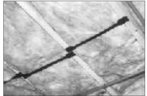
Figure 2. The ends of recycled-plastic Insul-Straps are wide enough for easy stapling. Insul Industries (2007 Yanceyville St., Suite 213, Greensboro, NC 27405; 800/372-7702) also makes a version with an adhesive strip on each tab for fastening to steel framing.
