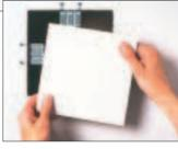
If you do much wall patching, you'll want to keep a supply of USG's new Drywall Repair Clips on hand. The clips make it easy to patch holes in drywall where there is no framing to fasten the
