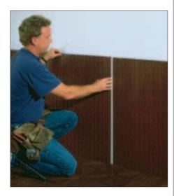
If you have a job that calls for simple, V-groove wainscot, then check out Wainscot Panels, a line of precut and prefinished veneer panels. The panels are 32 inches high (typical for wainscoting), and are finished with an acrylic topcoat. They come in wood veneer and simulated wood-grain styles. A small groove pattern is available in birch, cherry, oak, and pine; a wider groove pattern comes in birch, kaudamu, oak, and pine.
