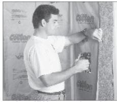
as a loose-fill blowing insulation for attics, and as traditional paper-faced batts. The material looks and feels like dryer lint, but insulates as well as fiberglass, doesn't cause itching, and requires no protective clothing or breathing devices during installation. The cotton insulation has code approval from SBCCI.
