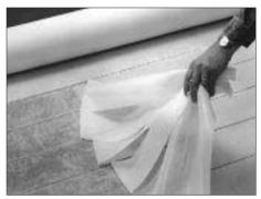
Hook-and-loop fasteners have been used on everything from sanding disks to sneakers. Now they've showed up on *TacFast*, a standard carpet bonded to a dense polyurethane foam cushion faced with a loop fabric. When you roll the carpet out, the loops catch on hook tape applied to the floor with pressure-sensitive adhesive, and hold the carpet in place.
