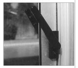
**B**arrier codes in some states require self-closing and self-latching doors on house walls that serve as one side of a pool enclosure. The intent is to keep small children from wandering out the door and falling into the pool. *Glidestar* is an automatic door closing and latching system for sliding doors. A weighted piston slides up and down a 1½- or 1½-inch-diameter aluminum tube mounted on the door stile. The piston
