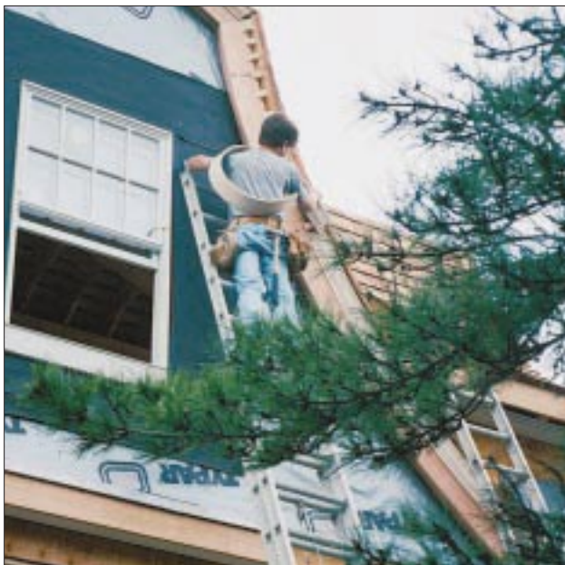
Figure 5. Special-order flexible molding saved the day when it came to trimming out the curved rakes. Angle blocks installed every few inches gave extra support to the floppy material.
