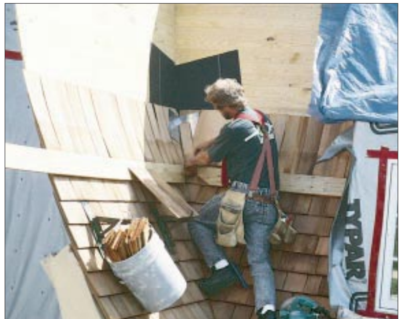
Figure 6. For extra protection at valleys, the roofer first installed a self-adhering membrane, then wove a piece of flashing into every course of shingles. The shingles were scribed tight to the valley.
