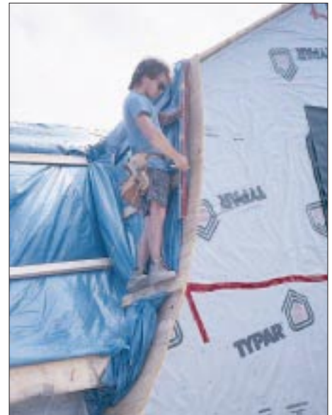
Figure 4. The author's crew used string and a level to mark the cut for the rake overhang on the curved roof sections.
