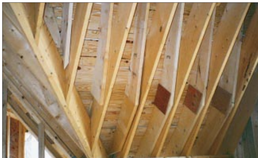
Figure 2. To frame the curves of the main gambrel, the author first installed a straight structural rafter on the inside, running from the purlin to the floor system. She then sistered two band-sawn 2x12s, spliced in the middle with a plywood gusset (see photo), to establish the curve on the outside of the roof.
