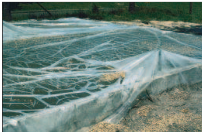
Figure 3. Besides compounds, other curing methods include sprinkling (left), which requires continuous monitoring, and poly (right), which is labor-intensive and may stain the slab.
