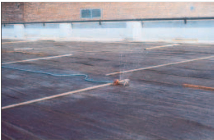
Figure 3. Besides compounds, other curing methods include sprinkling (left), which requires continuous monitoring, and poly (right), which is labor-intensive and may stain the slab.
