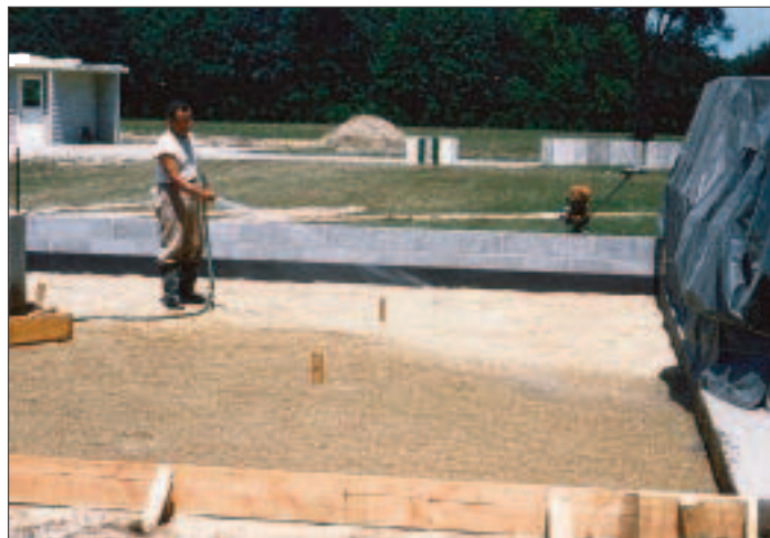
Figure 2. Wetting the subgrade before a pour prevents downward water migration, helping to keep slabs from cracking.
