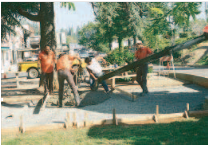
Figure 1. When pouring in hot weather, any slowdown will compound your problems, so have plenty of workers on hand.
