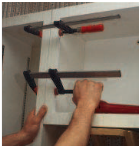
Figure 2. The author prefers Bessey bar clamps (left) for holding cabinets together. Quick-Grip Mini Bar Clamps (above) are useful where you must clamp one-handed. Because they lack the strength to lock the cabinets in place, however, the author uses them in combination with Bessey clamps.
