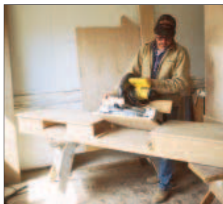
Figure 5. A homemade miter saw table is handy for solo trim cuts. The tabletop overhang provides a convenient surface for clamping jigs and stop blocks.
