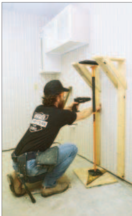
Figure 1. The author supports uppers with a pair of site-made brackets. He positions the top of the brackets a few inches below finish cabinet height, and uses shims and a T-Jak screw jack (shown leaning against the wall) to raise the cabinets to their final position.
