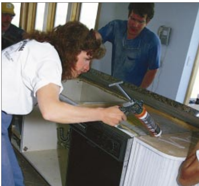
Figure 4. The author spreads silicone on the top of an end cabinet. The sealant is used more for uniform weight distribution than for adhesion — the stone's weight keeps it in place.
