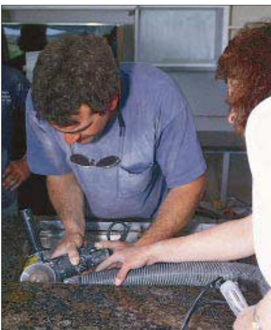
Figure 3. To avoid cracking granite counters during transport, the author waits to make sink cutouts until the slab is installed. She prepares the cutout in the shop by drilling holes at the corners and scoring the cut (upper left). She makes the final cut on site using a Skil 77 wormdrive saw fitted with a water shroud (upper right). The corners are cleaned up with a diamond blade on a grinder (lower left). With the cutout complete, sink installation is a straightforward task (lower right).
