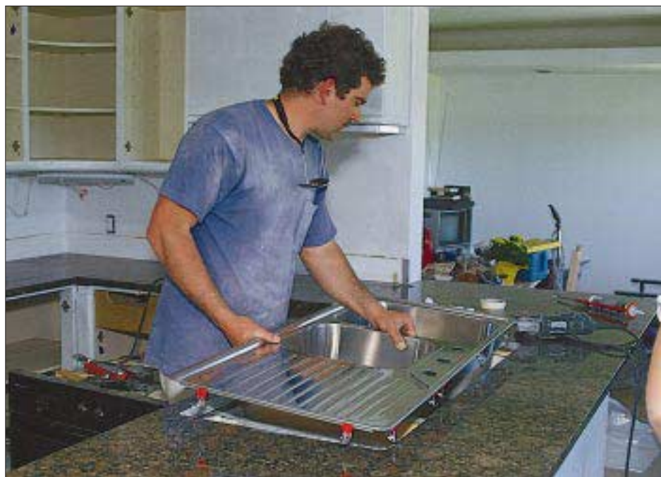
Figure 3. To avoid cracking granite counters during transport, the author waits to make sink cutouts until the slab is installed. She prepares the cutout in the shop by drilling holes at the corners and scoring the cut (upper left). She makes the final cut on site using a Skil 77 wormdrive saw fitted with a water shroud (upper right). The corners are cleaned up with a diamond blade on a grinder (lower left). With the cutout complete, sink installation is a straightforward task (lower right).
