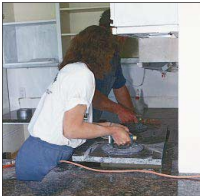
Figure 2 Suction cup handles, much like the ones used in the glass handling industry, make final positioning easier.
