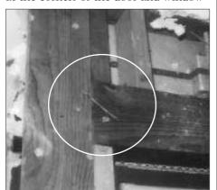
openings. During demolition, we found out why. When the house was built the framer installed what looks like a heavy gauge staple (about 6 inches long with 2-inch legs) at all joints between headers and king studs.
