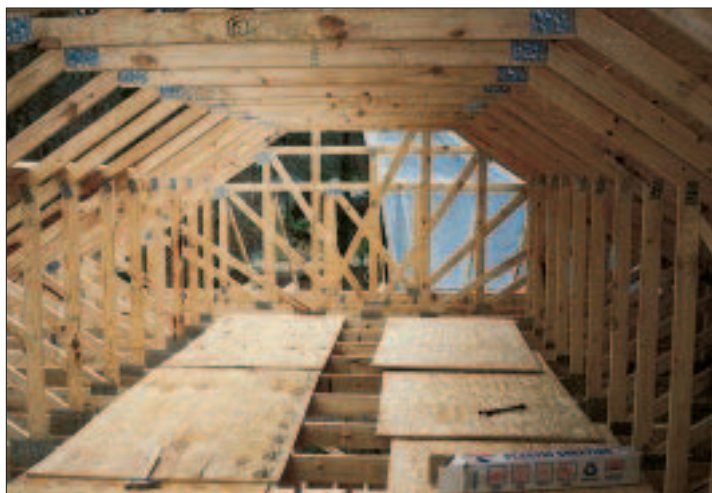
Figure 1. These storage trusses span 24 feet and provide a usable attic space 10 feet wide by 6 feet high.
