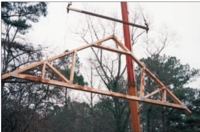
Figure 2. To minimize crane time, the trusses were lifted in bundles of three and placed on the third-floor wall plates.
