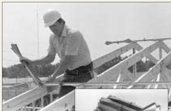
The Truslock spacing tool unfolds like a folding rule to maintain proper truss spacing.
