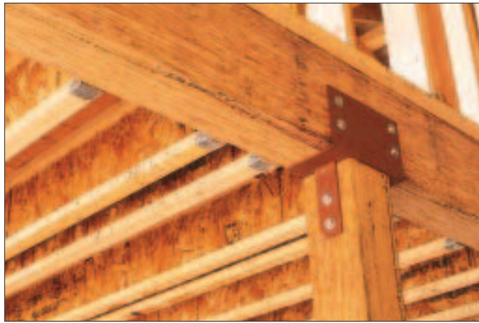
Steel connector manufacturers carry special hardware sizes to match the dimensions of engineered wood products like Parallam and I-joists. To avoid delays, be sure to order the connectors you need when you order the beams.
