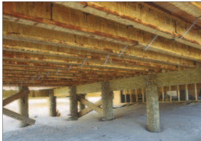
Parallam comes pressure-treated for exposed conditions. Recently treated beams may vary in size, but will eventually shrink back to the same dimension.
