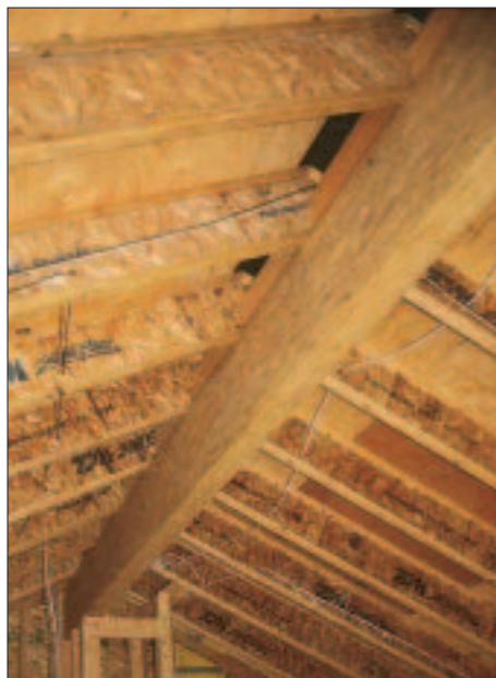
For a ridge beam, the author saves time by using a single piece of Parallam rather than laminating a multiple-member LVL beam.
