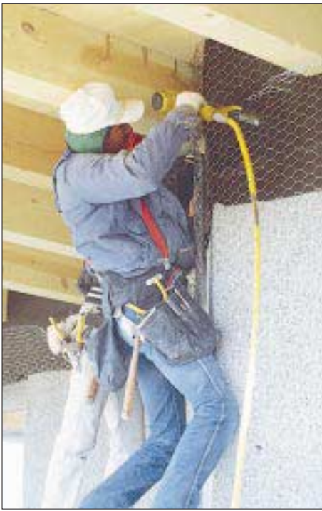
Figure 1. In preparation for one-coat stucco, a worker staples wire netting on wood-framed pony walls at the top of a masonry building.
