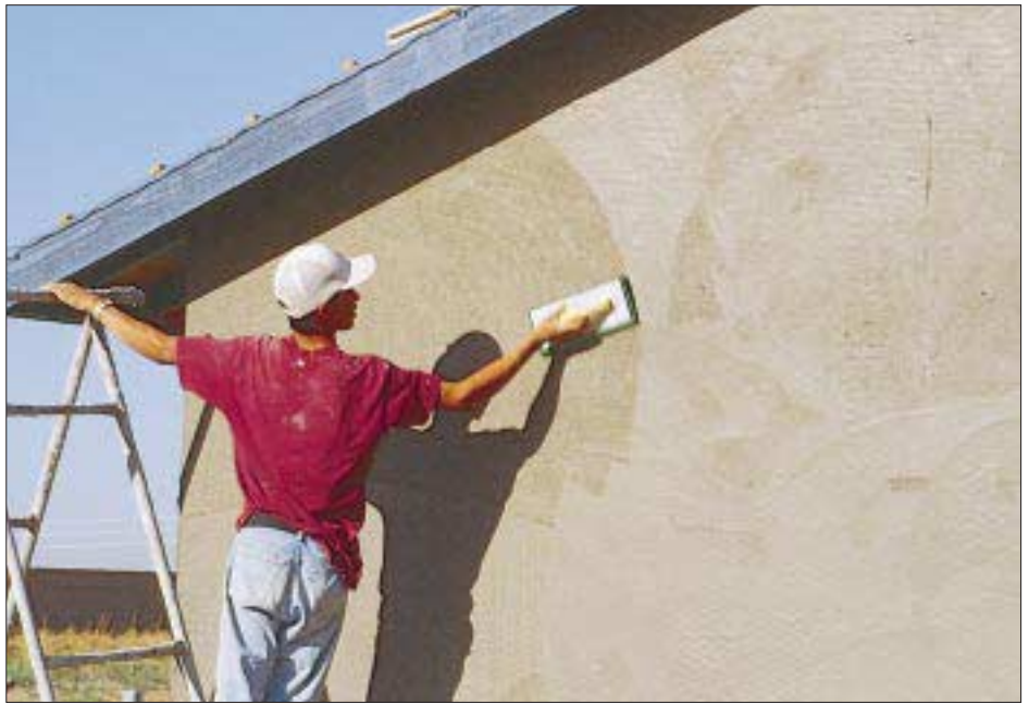
Figure 3. A worker smooths a cementitious base coat in preparation for a synthetic color coat.
