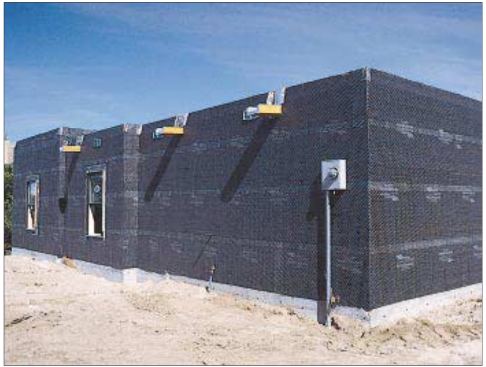
Figure 2. With wire netting installed over weather-resistive paper, this house is ready for stucco. Note the expanded metal lath around the windows and at the "canales," or rain scuppers, in the parapet walls.
