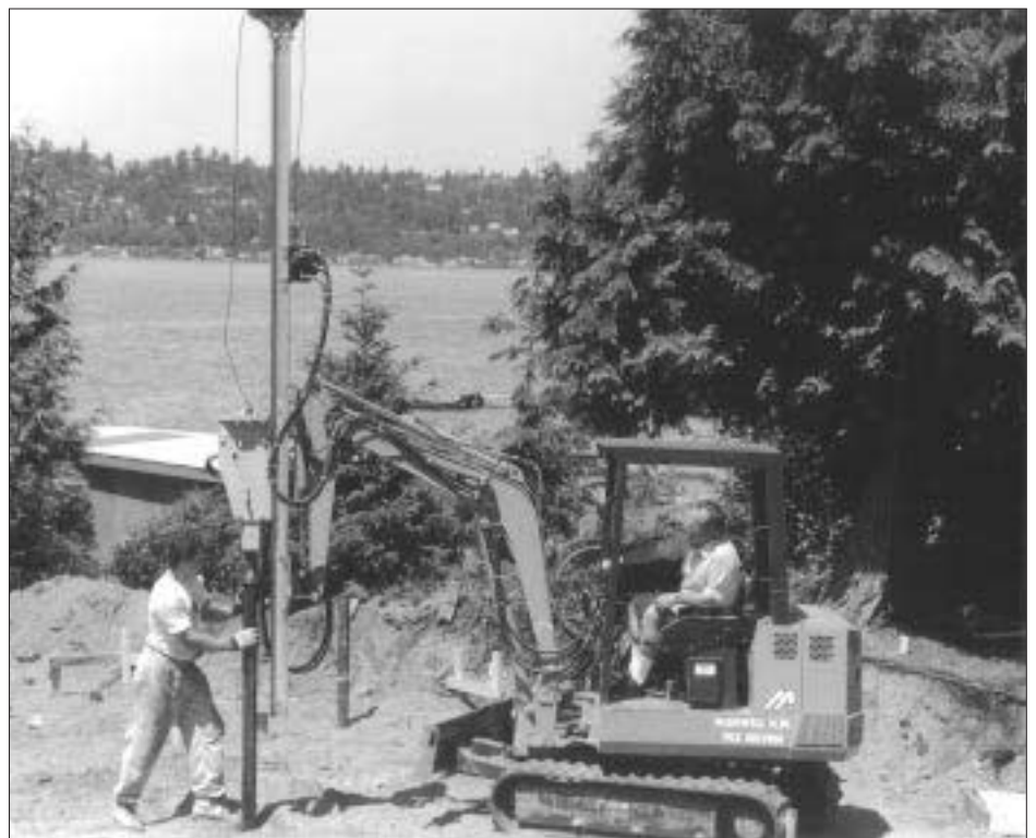
Figure 1. Pin piles are driven by a hydraulic hammer mounted on a small loader or backhoe.
