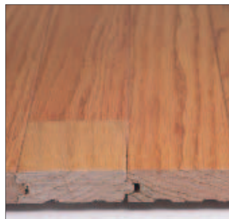
Figure 6. Many manufacturers reduce height discrepancies between adjacent floor boards by easing or V-grooving the edges.
