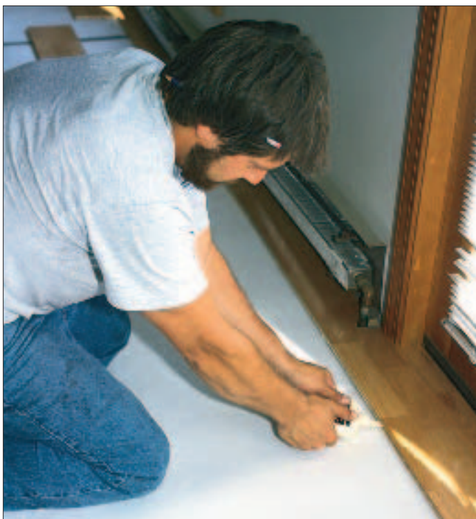
Figure 3. Instead of being fastened to the subfloor, most floating floors are installed by gluing adjacent boards to one another. The floor acts as a monolithic panel that's free to expand and contract.
