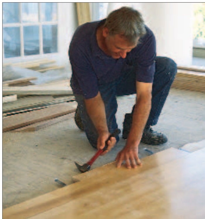
Figure 4. The only nonglued floating floor is made by Junckers. The boards are held in place with special metal clips.
