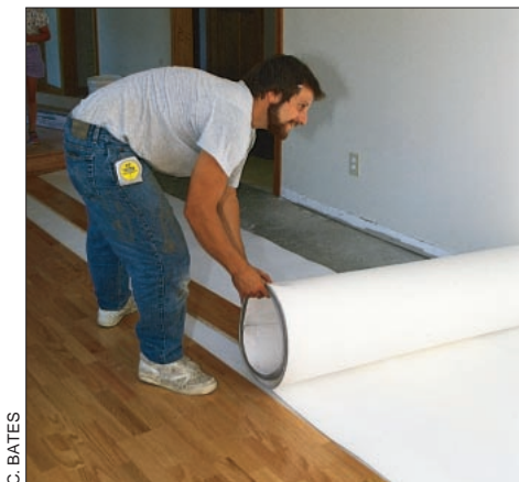
Figure 2. One advantage of a floating floor is that it can be installed over a continuous moisture barrier that doesn't get punctured by fasteners. A foam or felt pad must also be used as a gasket.
