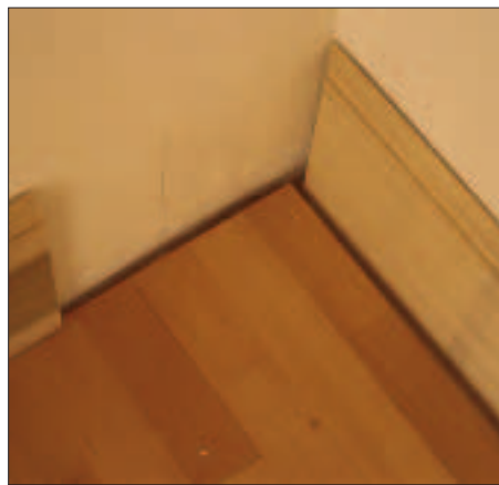
Figure 5. To prevent cracks from opening up between floor boards, the edges of a floating floor must have room to move freely with changes in temperature and moisture. A standard baseboard will cover the gap along the walls (left). At thresholds, some installers notch the ends into a tongue-and-groove header board that's fastened to the floor (right), but even this can restrain movement enough to cause problems.
