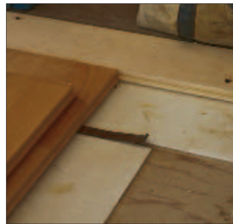
Figure 5. To prevent cracks from opening up between floor boards, the edges of a floating floor must have room to move freely with changes in temperature and moisture. A standard baseboard will cover the gap along the walls (left). At thresholds, some installers notch the ends into a tongue-and-groove header board that's fastened to the floor (right), but even this can restrain movement enough to cause problems.
