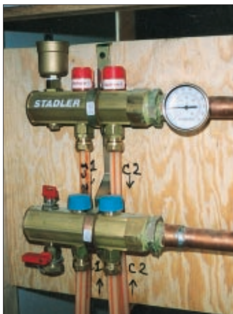
Figure 2. The four tubing circuits begin and end at a manifold station located in a wall inside a closet (left). Metal bend supports, supplied by the tubing manufacturer, protect the tubing from kinking as well as from the concrete finisher's trowels (right).
