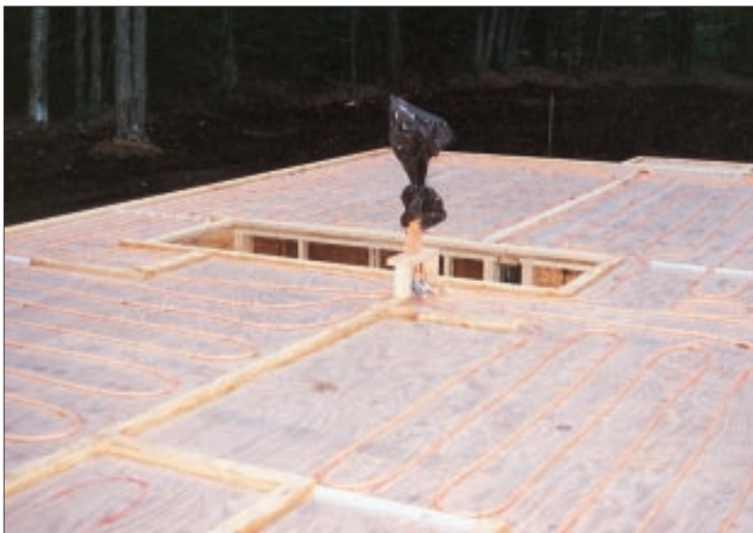
Figure 4. To prevent random cracking of the slab, control joints were created by nailing PVC drywall corner bead to the plywood subfloor (left). Control joints across doorways (right) and in the center of large rooms ensure that the slab cracks only in these locations.
