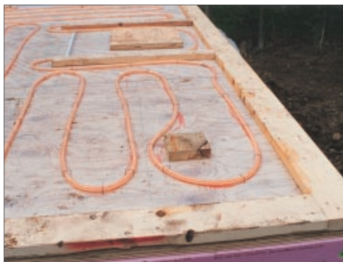
Figure 3. Prep for pouring the slab includes installing subplates for all the interior and exterior walls, and blocking for the toilet flange and other mechanicals.
