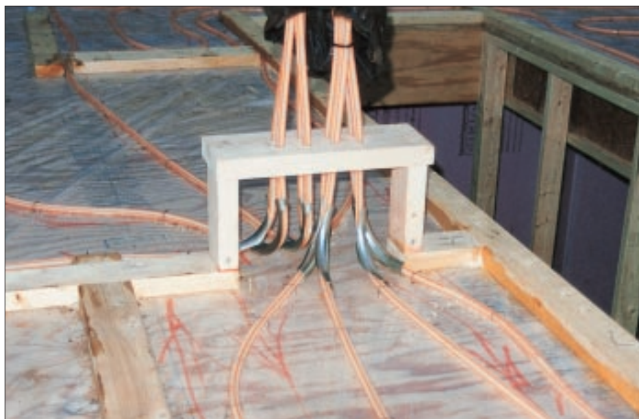
Figure 2. The four tubing circuits begin and end at a manifold station located in a wall inside a closet (left). Metal bend supports, supplied by the tubing manufacturer, protect the tubing from kinking as well as from the concrete finisher's trowels (right).
