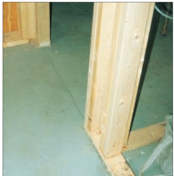
Figure 4. To prevent random cracking of the slab, control joints were created by nailing PVC drywall corner bead to the plywood subfloor (left). Control joints across doorways (right) and in the center of large rooms ensure that the slab cracks only in these locations.
