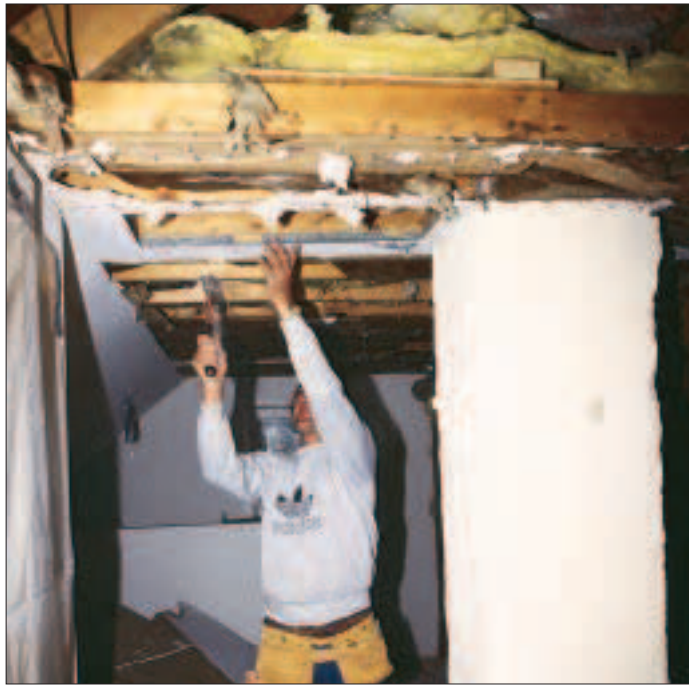
Figure 1. As demo proceeds inside the house (top), carpenters strip shingles on the outside (middle). A hole opened up in one end of the roof allows demo debris from inside to be tossed directly into the dumpster (bottom).
