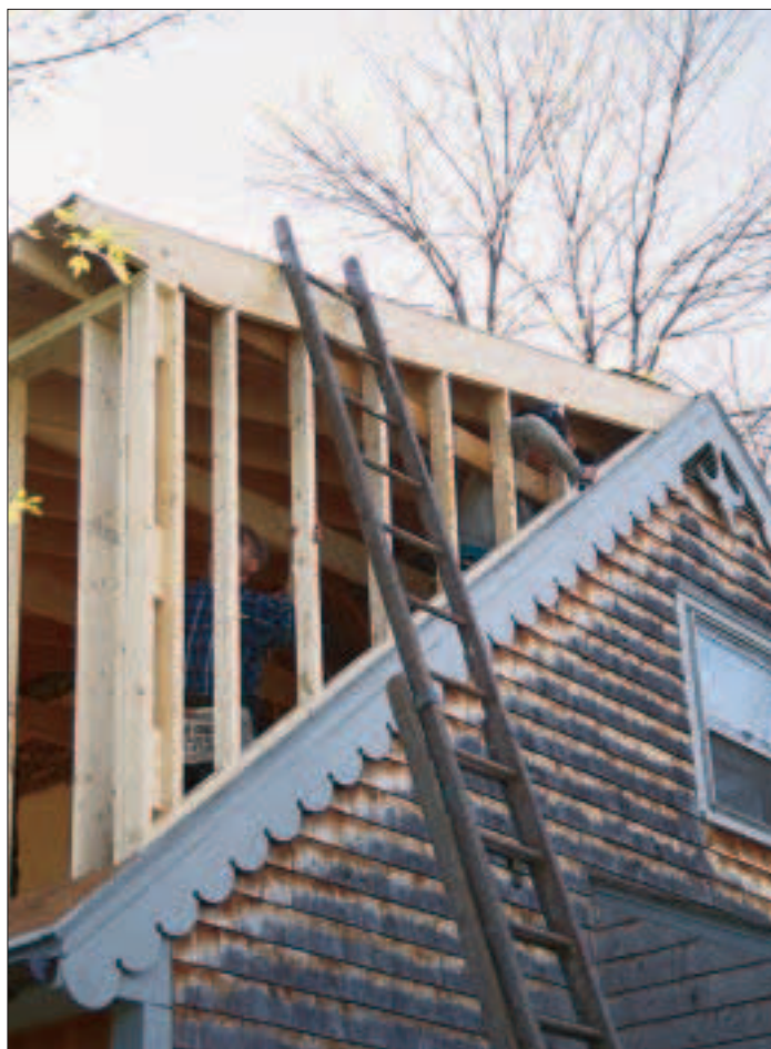
Figure 5. By the end of the second day, the dormer roof is sheathed and papered (left). The finished dormer maintains the low-profile look and feel of the original cape (below).
