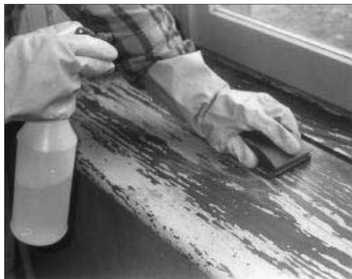
Figure 1. Chemically stripping painted woodwork (left) is a safer alternative than sanding. If you must sand, wet the woodwork to keep dust levels down (right), then repaint with a high-quality oil/alkyd for maximum protection.
