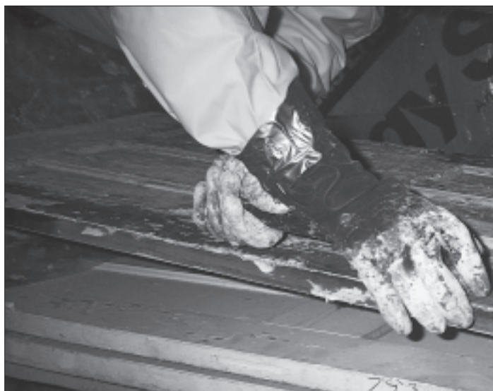
Figure 1. Chemically stripping painted woodwork (left) is a safer alternative than sanding. If you must sand, wet the woodwork to keep dust levels down (right), then repaint with a high-quality oil/alkyd for maximum protection.
