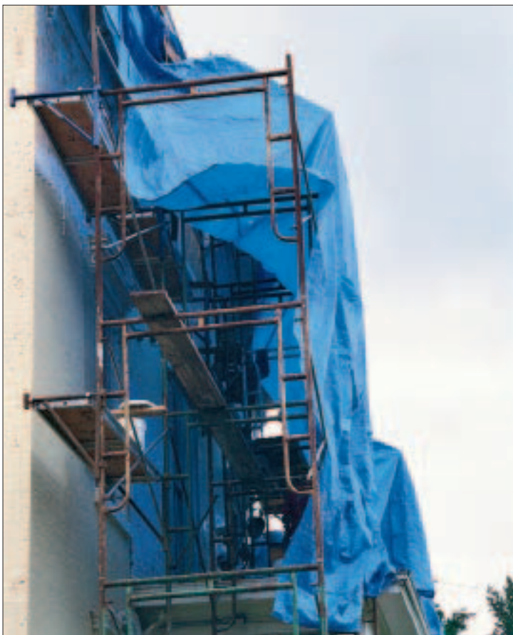
Figure 2. When sanding or water blasting a house exterior, shroud the scaffolding with plastic or tarps to contain dust and overspray.
