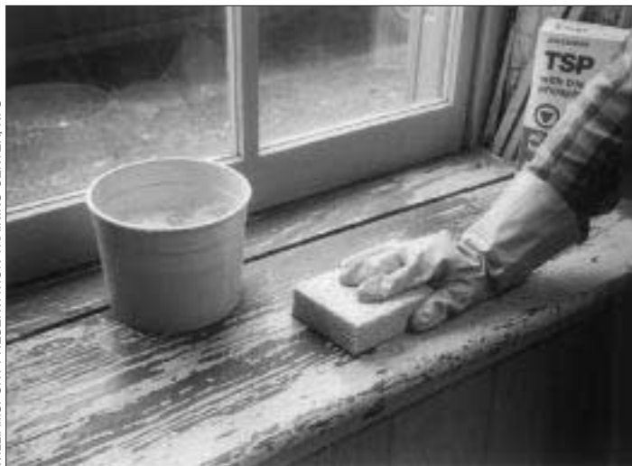
Figure 3. Job-site cleanup includes washing down walls and woodwork with a phosphate solution, such as TSP, or a detergent containing EDTA.
