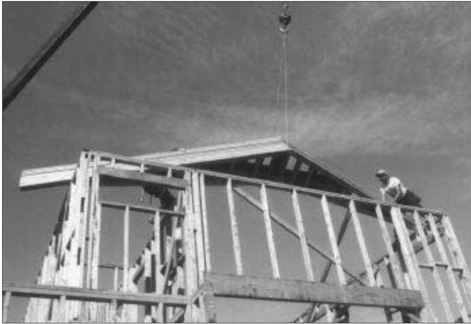
Figure 1. To get the job underway, the crane first sets a bundle of trusses near one end of the building, resting them across the two sidewalls and the gable-end wall (left). The carpenters then spread the trusses evenly across the walls, starting at the opposite end and working back (right).
