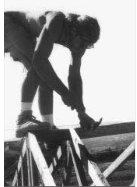
Figure 3. Installing the supplied blocking as each truss is set automatically maintains the proper spacing — although on-center dimensions should be verified every few trusses. The author's crew always installs plate blocks first (left), then goes back to install ridge blocking (right).
