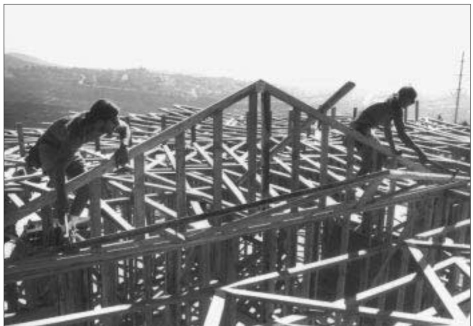
Figure 2. Truss roof framing typically starts with a gable-end truss, recognizable by the vertical members.
