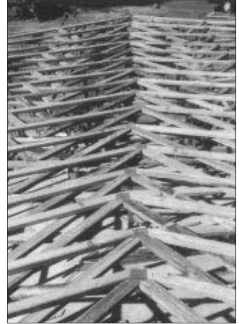
Figure 1. To get the job underway, the crane first sets a bundle of trusses near one end of the building, resting them across the two sidewalls and the gable-end wall (left). The carpenters then spread the trusses evenly across the walls, starting at the opposite end and working back (right).
