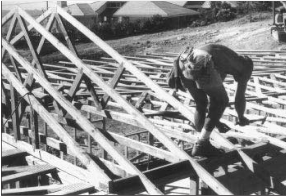
Figure 3. Installing the supplied blocking as each truss is set automatically maintains the proper spacing — although on-center dimensions should be verified every few trusses. The author's crew always installs plate blocks first (left), then goes back to install ridge blocking (right).
