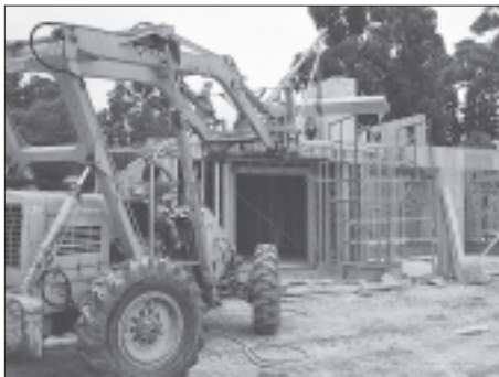
Figure 3. To reduce time lost handling materials, the author sometimes uses a Pettibone or forklift as a storage platform or to hoist materials onto a roof or second story.
