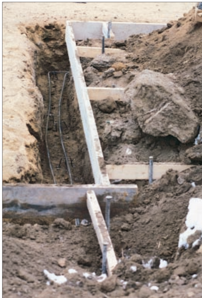
Figure 2. Because the trench walls are often too unstable to hold stakes, the author hangs the slab form boards over the trench with horizontal 2-by braces spaced 4 feet apart. To keep the braces out of the way during the pour, position them flush or below the top of the form board.
