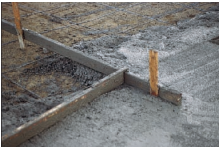
Figure 4. With the bottom of the interior 2x4 screed set to finish slab height, a 1x2 "hook" attached to a 2x4 drag board will ride on top of the screed. The bottom of the other end of the drag board rides on the perimeter form.
