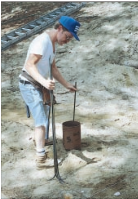
Figure 4. Rebar goes in when the tube is partially full of concrete. The bend at the end of the rebar ties the pier to the footing.
