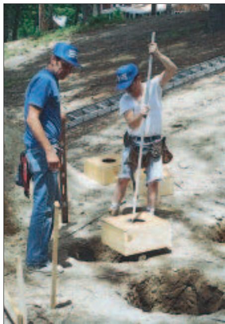
Figure 2. The author makes pier footing forms from scrap lumber and plywood and lowers them into the hole with a hoe.
