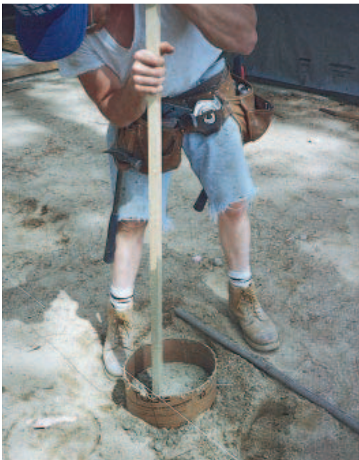
Figure 5. Tamping throughout the pour gets rid of voids in the pier. The nail in the side of the tube marks the finish concrete elevation.
