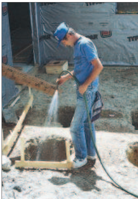
Figure 1. Saturating the pier hole with a garden hose helps compact the soil at the base to keep it from settling.
