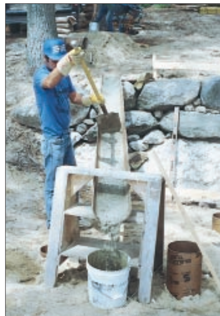
Figure 3. When mixing concrete by hand, a tube ripped in half with a circular saw makes a convenient chute.
