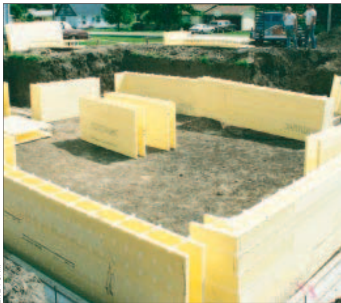
Figure 4. To speed construction, the author preassembles Lite-Form panels into 8-foot-high wall and corner sections up to 16 feet long. Starting at the corners, the panels are set against a 2x4 kicker nailed to the footing.
