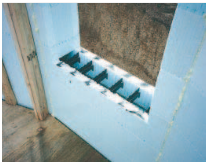
Figure 8. End caps slipped into the dovetail grooves on the inside face of the blocks create a bulkhead at wall drops and window and door openings.
