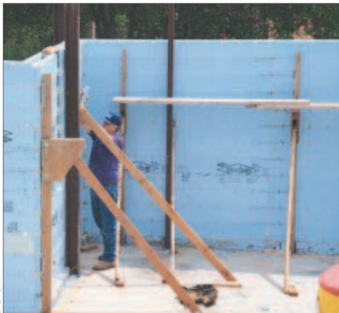
Figure 5. The foam forms are braced with vertical 2x4s fastened to the wall ties with angle brackets and screws. Plywood gussets hold 2x12 planks that both stiffen the wall and provide scaffolding during the pour. Note the mason's line "stitching" the form sections together.
