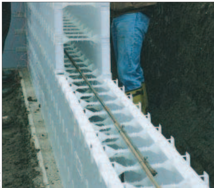
Figure 3. Heavy-duty plastic ties are critical to the Lite-Form foam panel system: They connect the panel ends, support the rebar, and hold the panels together during the pour. Because the plastic is so dense, the ties also provide a nailer for drywall and siding.
