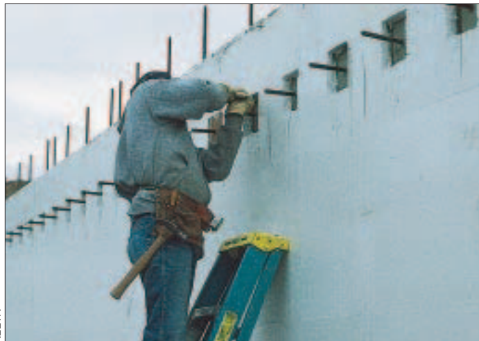
Figure 2. Ledgers for the floor systems are fastened to concrete bond beams in the wall. After the concrete hardens, treated-wood spacers are inserted into holes cut in the foam to keep the ledger from crushing the foam.
