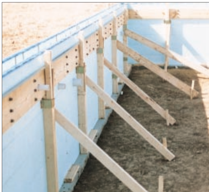
Figure 7. Lumber braces on 6-foot centers support the floor ledgers, with anchor bolts in place, until the concrete is poured. The vertical bracing also serves to support scaffolding brackets.
