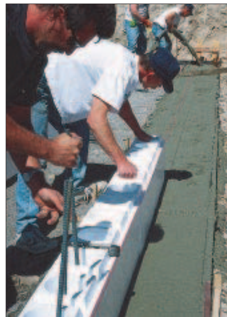
Figure 1. On the first day, the crew pours the footing, embeds the first course of Keeva blocks in the wet concrete, and sets the vertical rebar hooks. Once the starter course is set, the crew can lay 1,200 to 1,500 square feet of wall per day. Concrete poured into selected cells results in a concrete post-and-beam structure, with columns on 8-, 16-, or 24-inch centers.
