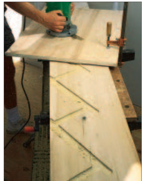
Figure 3. Because the router's guide bushing is wider than the bit, the template must be wider than the channels to be routed in the stringer. To help with alignment, the bottom of the template is covered with 1/4-inch plywood: The cutout in the 1/4-inch plywood matches the channel in the stringer. With the treads and risers marked, the template is slid up and down the stringer (photo, right). The guide strips on the underside keep it centered.
