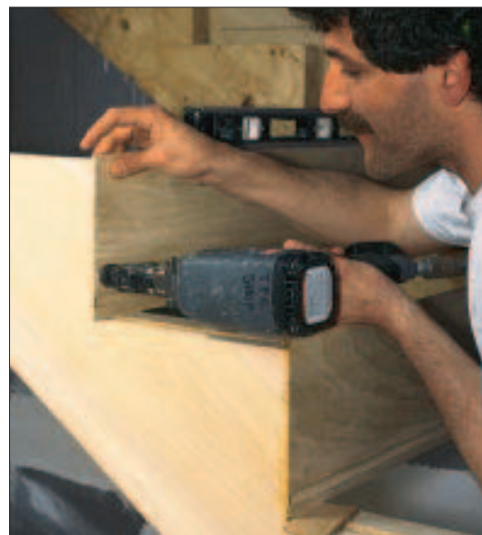
Figure 6. With one end of the riser temporarily shimmed to the closed stringer, the riser is leveled and fastened to the open stringer.
