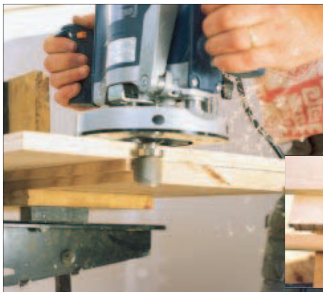
Figure 7. To finish the end cut on the tread, the author uses a plywood template and a flush-cut bearing bit. The inside corner of the nosing is sanded to match the slightly rounded cut on the tread.
