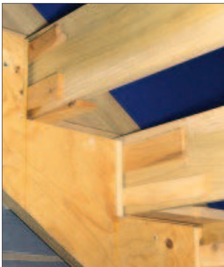
Figure 4. To make it easy to install the risers, the author positions the finish stringers so that the plumb cuts are slightly forward of the plumb cuts in the rough carriages. He then shims the risers to the rough carriage.
