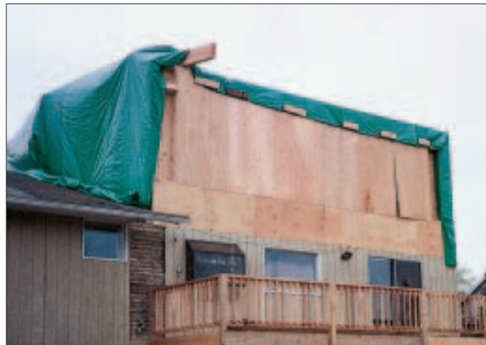
Figure 1. To prevent the tarp from ripping, the author secures it to the building with nailed 2x4 blocks.
