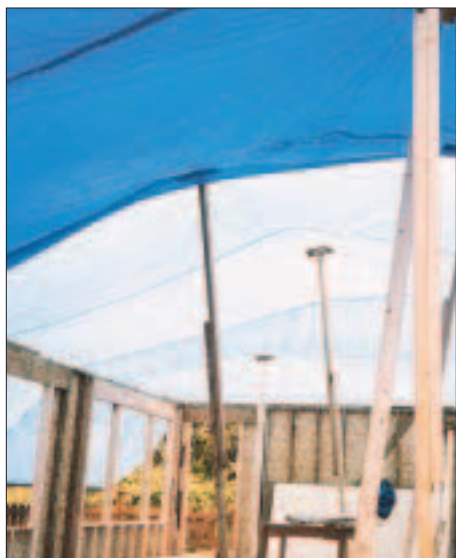
Figure 2. Long vertical supports, or “taut sticks,” made of spliced-together 2x4s create a dry, roomy work space on rainy days.
