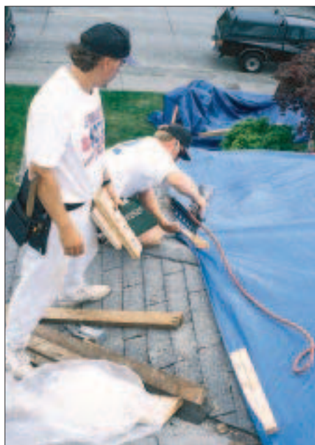
Figure 3. For efficiency, the author’s crew works in two-person teams. Here, the lead man pulls the tarp tight and secures it while the support man passes him the nail gun and blocks as he needs them.
