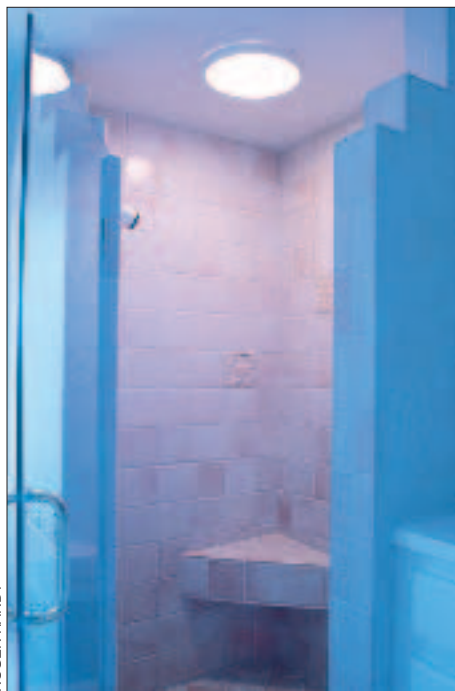
Figure 2. Whenever there's room, the author includes a bench in the shower for the bather to sit on while washing feet or shaving legs. This triangular corner bench is easy to frame and looks good.
