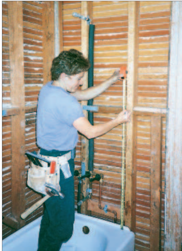
A carpenter marks the location for securing a vertical grab bar into the framing. Note the height of the showerhead stub — at 84 inches off the subfloor, it allows room for bathers taller than 6 feet.
