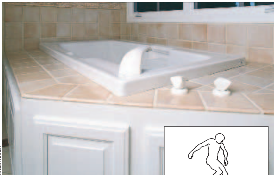
Figure 3. Elevated, sunken tubs are hard to get into safely (right). The author avoids steps and provides a wide ledge next to the tub (above). Users can then safely sit on the tub ledge and swing their legs into the tub.
