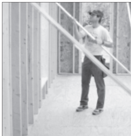
Nate Seymour of Hagstrom Contracting brings a wall in line with a quick twist of a Proctor wall brace.
