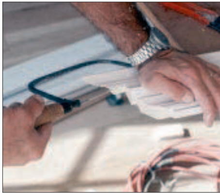
Figure 2. Three ways to cope crown: In the hands of a seasoned carpenter, a coping saw (left) can cut with amazing speed and accuracy. Another carpenter prefers a jigsaw to remove the bulk of the material along the molding's profile (center). Then to smooth out the cut to a perfect feather edge, he uses a mini-grinder with 60-grit paper (right).
