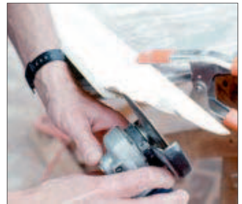
Figure 2. Three ways to cope crown: In the hands of a seasoned carpenter, a coping saw (left) can cut with amazing speed and accuracy. Another carpenter prefers a jigsaw to remove the bulk of the material along the molding's profile (center). Then to smooth out the cut to a perfect feather edge, he uses a mini-grinder with 60-grit paper (right).
