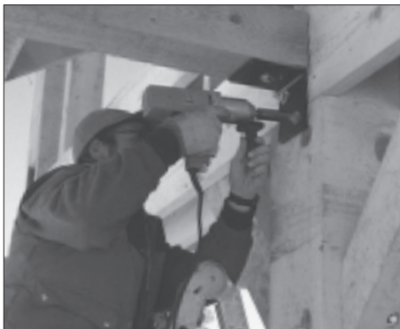
An electric impact wrench can "hammer" long lags or heavy machine bolts into place without transferring much torque to the handle or stalling the motor.
