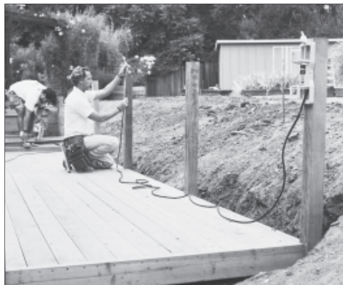
A water level, such as this Zircon Pro Series, quickly establishes a level plane. Here it is used to mark the top cut on some deck posts.
