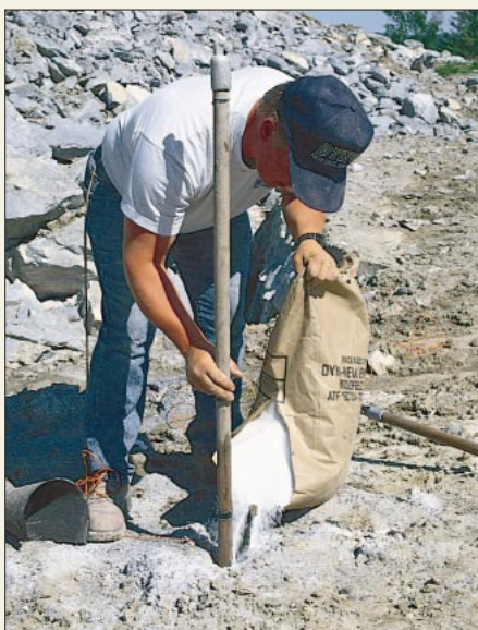
The author uses nonelectric blasting caps and fuses because they cannot be triggered by radio waves (left). Bagged nitrate poured down the bore hole on top of the dynamite is an inexpensive but powerful explosive (right).
