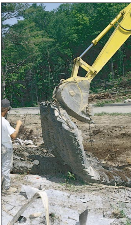
Figure 1. To protect nearby houses from flying debris, an excavator places protective mats over the blast site.
