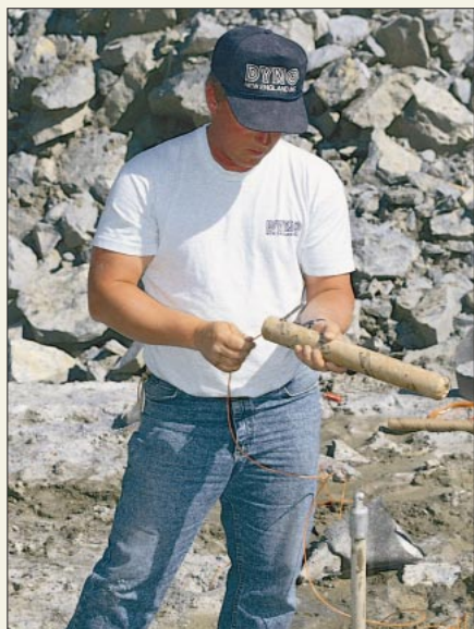
The author uses nonelectric blasting caps and fuses because they cannot be triggered by radio waves (left). Bagged nitrate poured down the bore hole on top of the dynamite is an inexpensive but powerful explosive (right).
