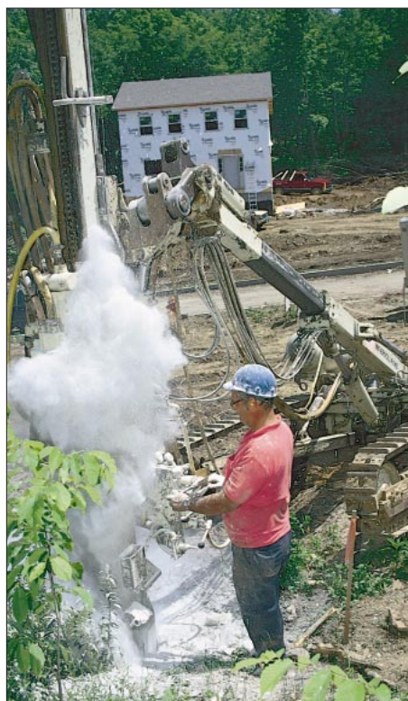
Figure 2. A track-mounted drill can quickly and easily locate all the rock on the site.
