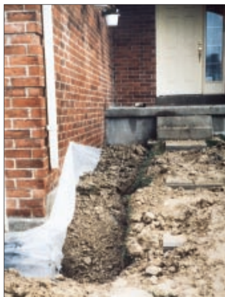
Figure 2. Unheated garages are prone to damage from adfreezing (left). Two layers of 6-mil polyethylene placed on both sides of the foundation wall provides a slip plane that prevents freezing soils from bonding to the foundation wall (right).
