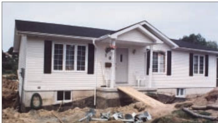
Figure 3. The foundation of this factory home (left) was built on unstable soil. Settlement caused extensive foundation damage (middle), which required complete excavation and engineered underpinnings (bottom).
