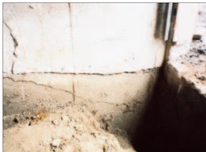
Figure 1. As the soil around an unheated building freezes and expands, it can “grip” the foundation and lift the wall apart (left). Although block walls are particularly susceptible, poured concrete walls can also be damaged (above).
