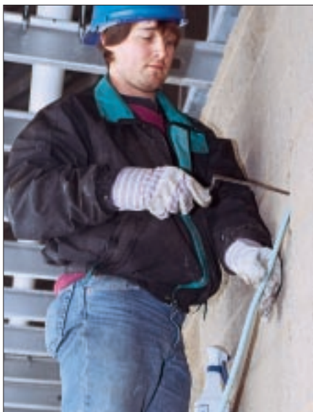
Figure 2. Compressible foam backer rod fills the back of a joint and helps the caulk perform properly. Use a size slightly thicker than the crack and insert it gently with a blunt tool.
