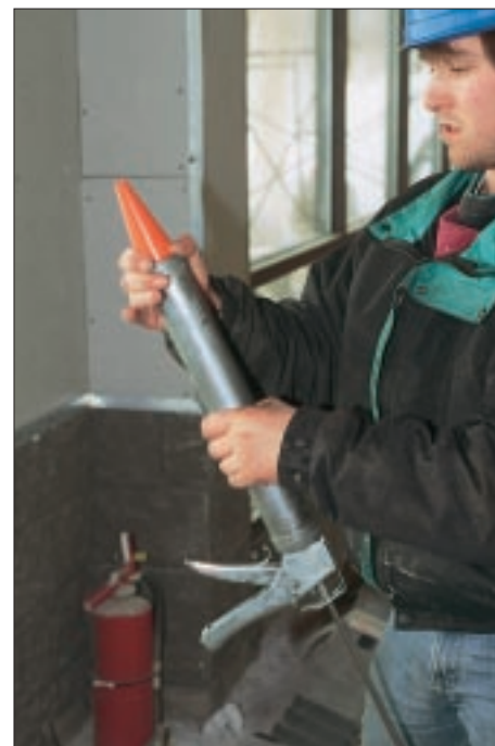
Figure 1. Two-part bulk sealants have to be mixed with a drill and paddle (left). Using a bulk caulking gun (middle and right) allows you to do high-volume caulking more cost-effectively, but is messy.
