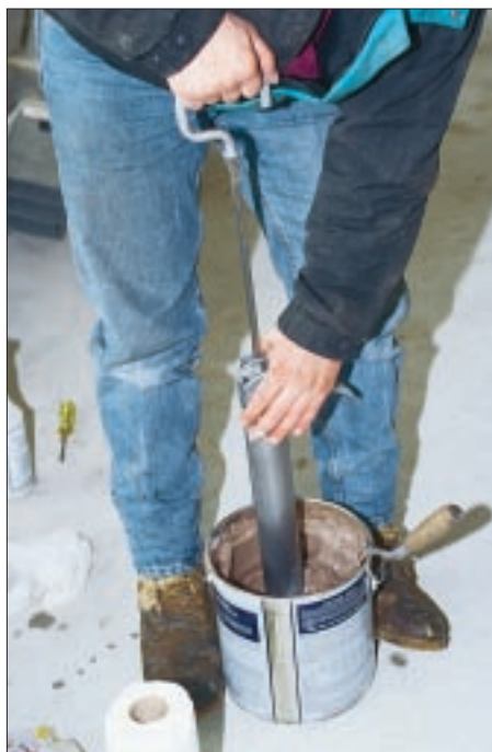
Figure 1. Two-part bulk sealants have to be mixed with a drill and paddle (left). Using a bulk caulking gun (middle and right) allows you to do high-volume caulking more cost-effectively, but is messy.
