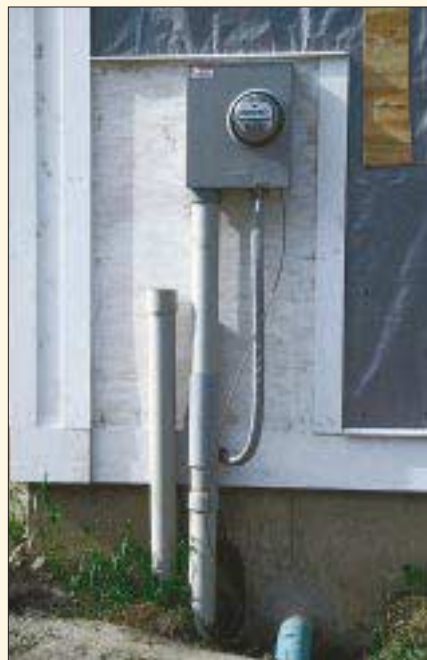
Figure A. The PVC riser that carries the main service feed to a house's electric meter needs an expansion fitting near the ground. Without it, the movement from the freezing and thawing of the soil could crack the pipe.
