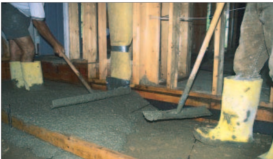
Figure 3. Here, 3-inch strips of asphalt-impregnated expansion board isolate a slab from wood framing. The flatworkers can also use the expansion board as a guide for finished slab height.
