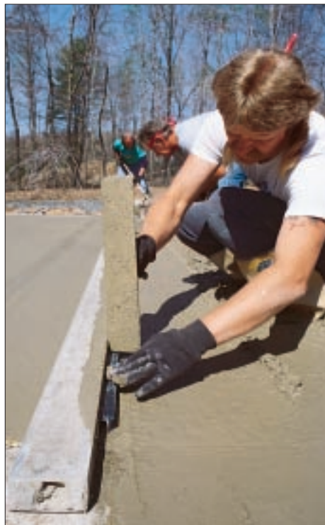
Figure 6. Two-piece plastic control joint materials are popular on residential sites. The tee-shaped extrusion is pressed into the wet concrete (left), then the top, horizontal piece is "zipped" off, leaving an invisible control joint (right).
