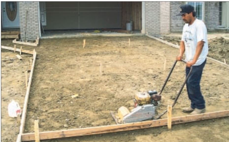
Figure 1. To prevent settlement cracks, the subgrade must be compacted properly. Here, a worker uses a vibratory plate compactor to correctly prepare the subgrade.
