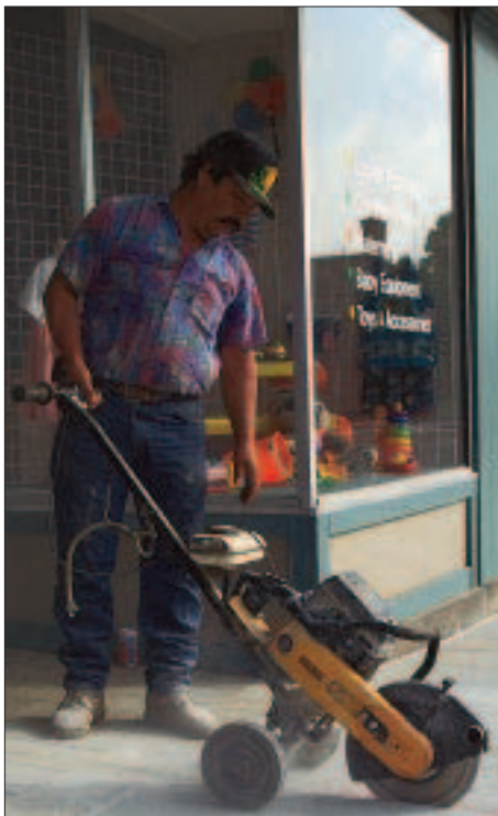
Figure 5. Sawn joints are cut with a power saw equipped with a diamond blade. They should be cut soon after the surface hardens.
