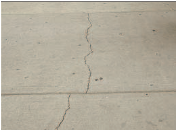
Figure 7. Rectangular slabs tend to crack in the middle. Control joint spacing should equal slab width.
