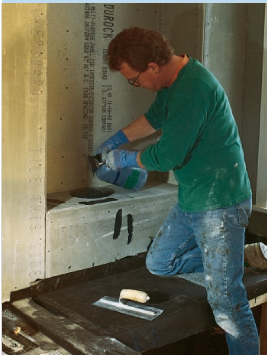
The author applies a two-part waterproofing membrane to tile backerboard in a steam room installation.
