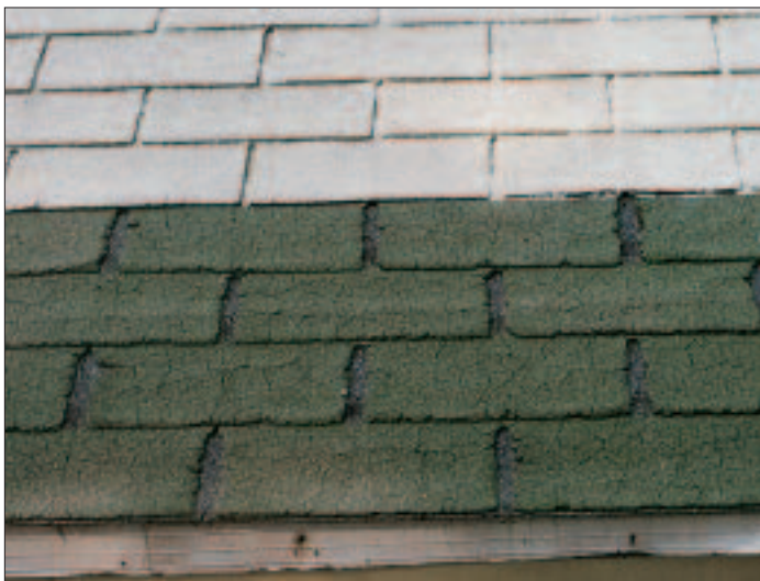
Shingles deteriorate badly over time, but a pigmented elastomeric acrylic coating can give many years of protection.
