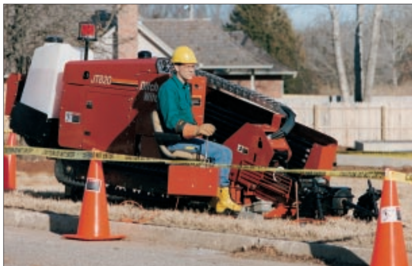
New equipment like this Ditch Witch model JT820, introduced in 1995, can drill holes through soil or rock for utility lines without disturbing the landscape surface.
