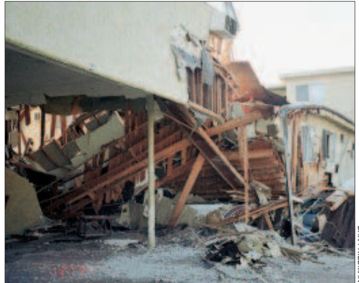
Earthquake damage like this could be prevented with a structural retrofit costing a few thousand dollars per apartment, say Los Angeles engineers.
