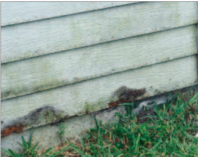
Hardboard siding exposed to moisture sometimes deteriorates. Manufacturers blame faulty installation and maintenance, but attorneys suing the companies say the siding material itself is defective.
