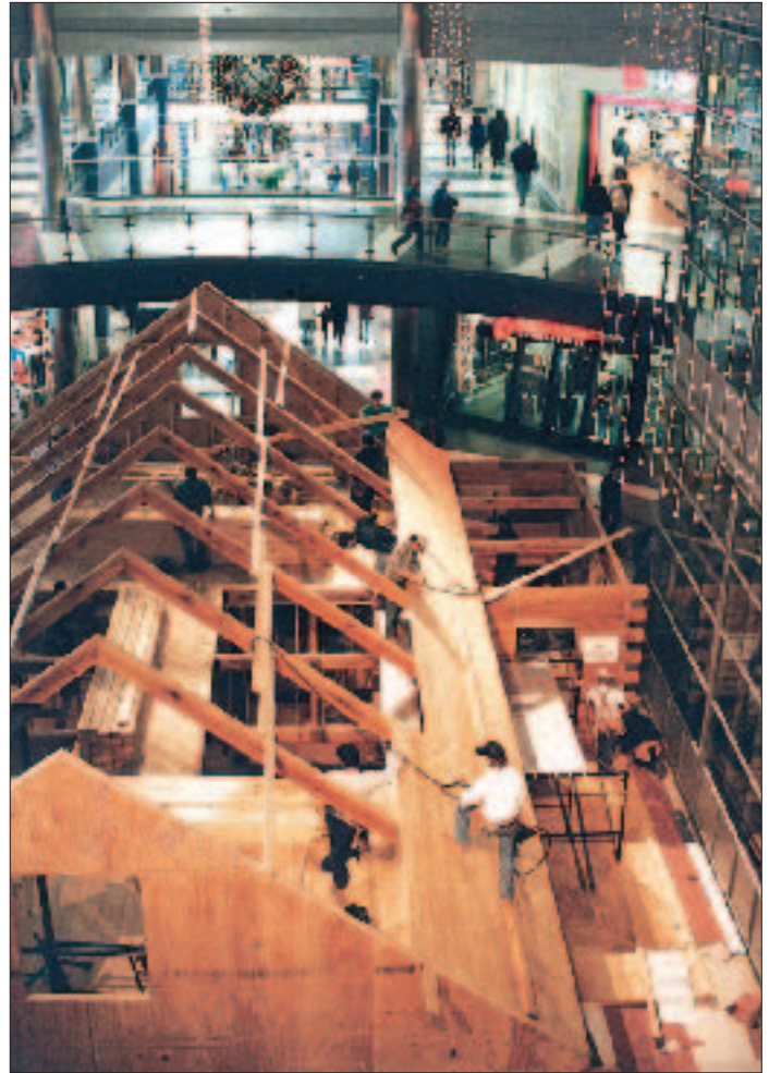
Gastineau Homes (800/653-6533) erected this log home package inside the Mall of America in Minneapolis, Minn.
