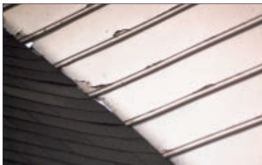
Edge swelling and dimpling around nails are common hardboard complaints (above left). Sometimes, severe deterioration follows: A Baltimore-area home inspector was able to poke his finger through rotting hardboard siding (above). Installation details can contribute to problems: The hardboard shown at left was placed in direct contact with a roof surface, contrary to manufacturer instructions.
