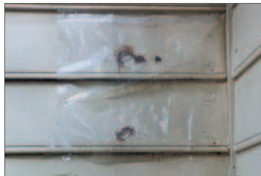
Edge swelling and dimpling around nails are common hardboard complaints (above left). Sometimes, severe deterioration follows: A Baltimore-area home inspector was able to poke his finger through rotting hardboard siding (above). Installation details can contribute to problems: The hardboard shown at left was placed in direct contact with a roof surface, contrary to manufacturer instructions.
