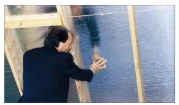
Radiant barrier attic sheathing keeps a hot roof from radiating heat to the ceiling and ductwork below. In an Austin, Texas, test, the material cut home cooling needs by 16%.
