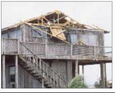
Metal roofs like the one shown, and many asphalt shingle roofs, suffered blow-offs in the storm (above). Some gable end trusses failed when 80-mph to 100-mph winds tore sheathing off roof edges, leading to partial roof collapses (left).
