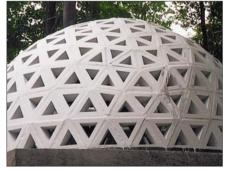
Using an innovative triangular block mass-produced at a local block plant, students from Alfred State College assemble a prototype geodesic dome. The system's inventor says half-triangle blocks can be used to create square openings for standard windows and doors.
